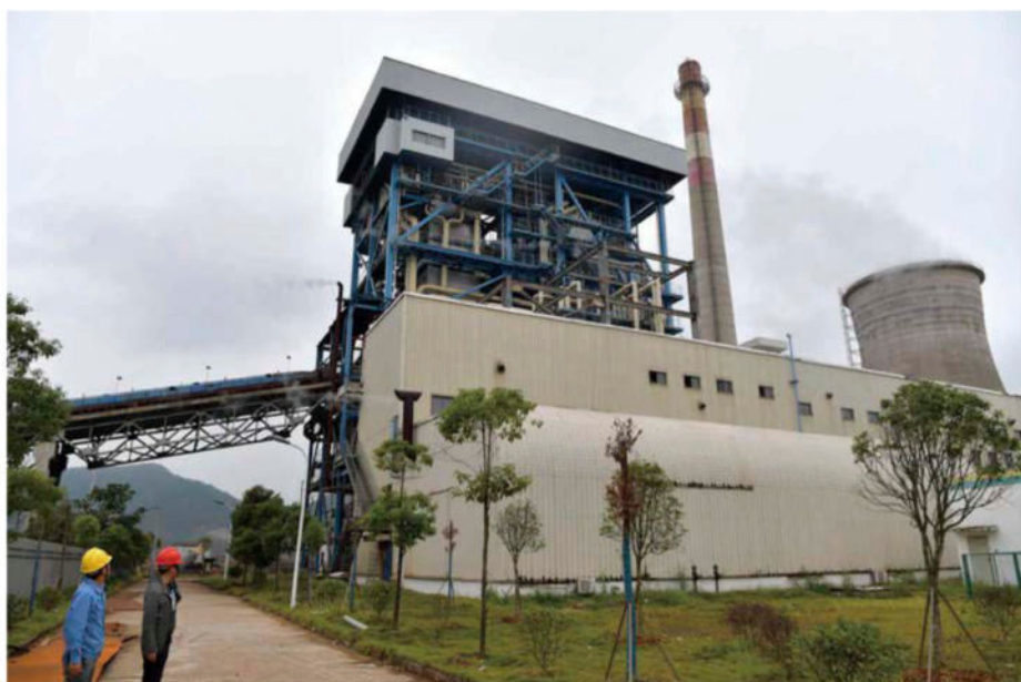
A power plant in Yongxin County, east China's Jiangxi Province
