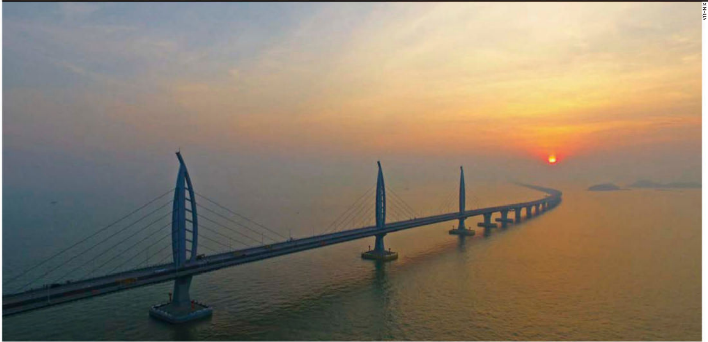
The Hong Kong-Zhuhai-Macao Bridge on December 31, 2017
